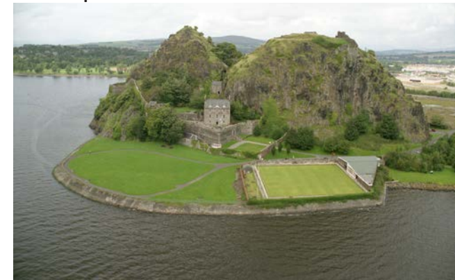
The Bowling Green is important part of the site
