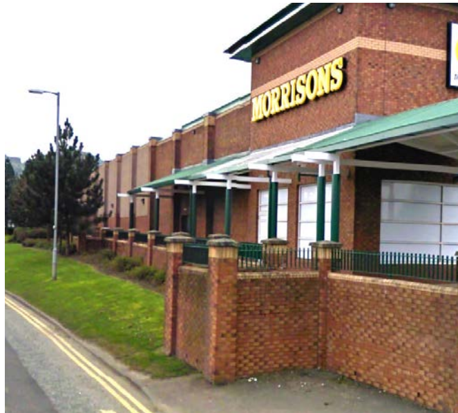
A Route from Morrison's has been blocked
