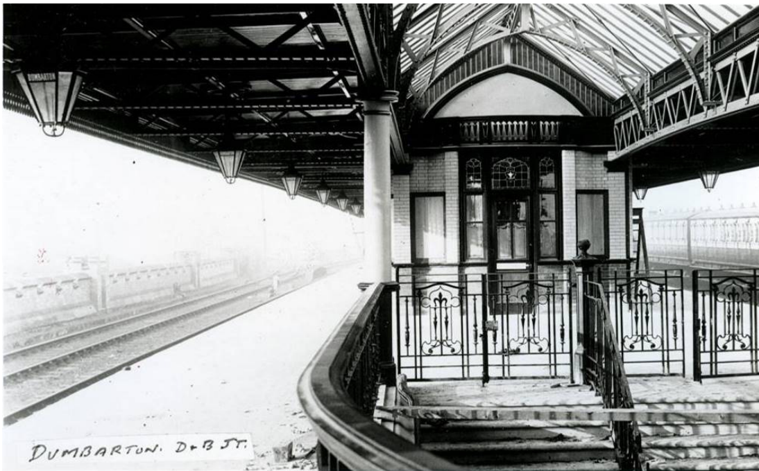
Figure 26 c.1935 image of the south platform of Dumbarton Central Station showing the former hanging lanterns labelled with 'Dumbarton' and the now-enclosed south stair and decorative wrought iron gates. 73
