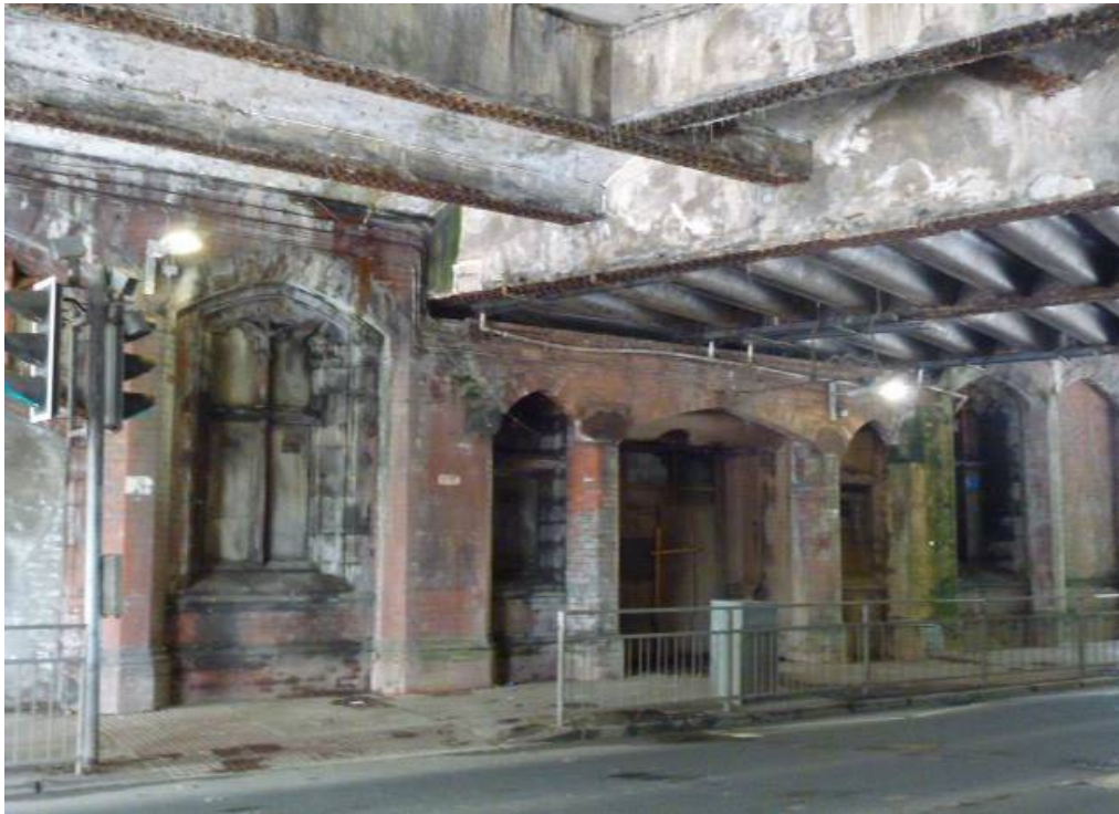
Church St. elevation and bridge deck (2018)
