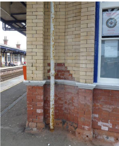
Figure 45 Inappropriate repairs - injected chemical DPC (L) and Non-matching brick replacements & loss of detail at Station Road (R)
