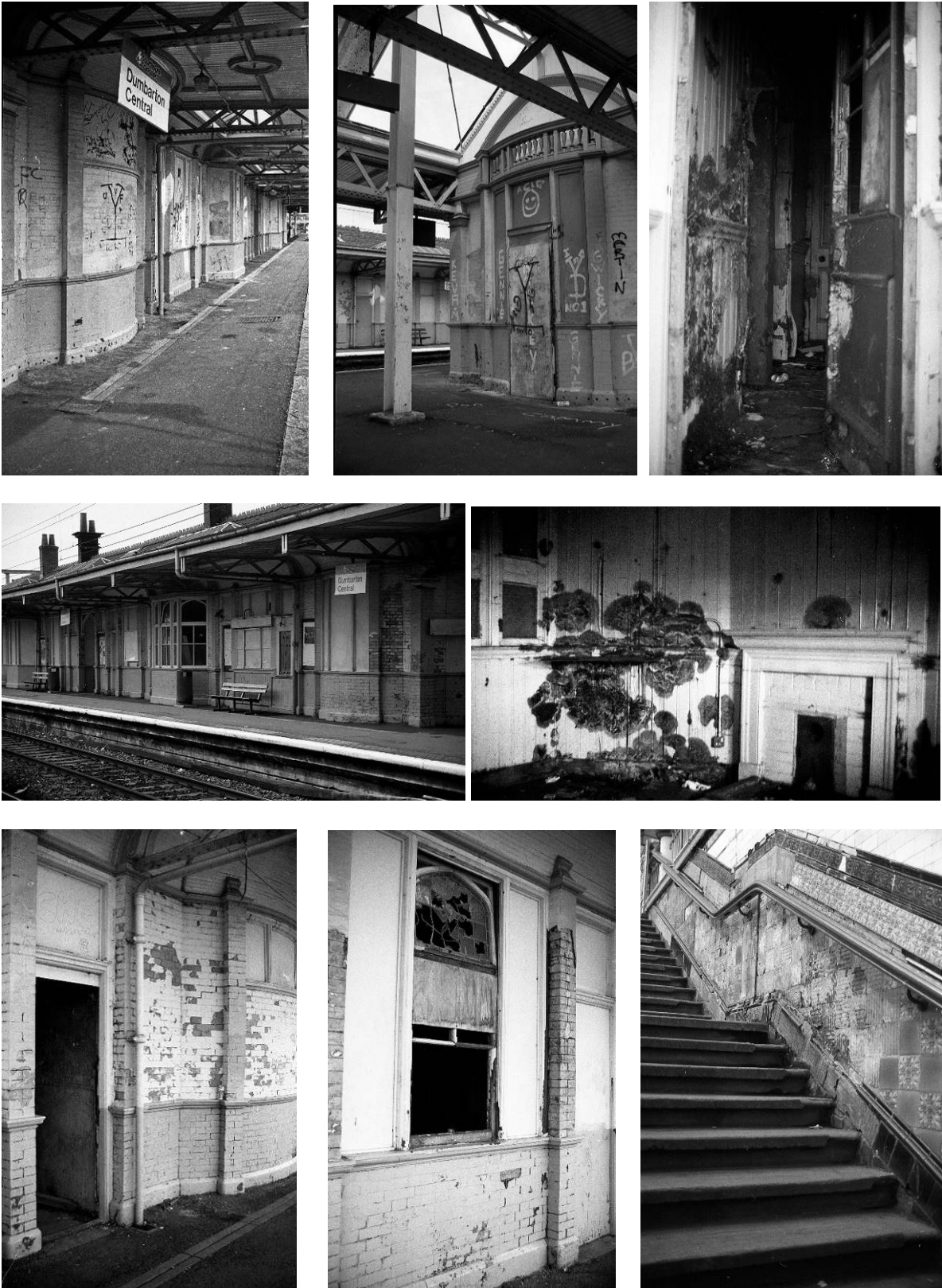
Figure 37 Photographs taken in 1989 showing the derelict state of the station at this time prior to refurbishment works. 82
