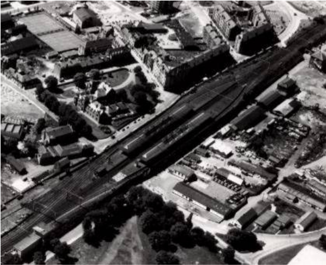
Figure 30 Aerial photograph looking southwest taken in 1973 77 showing new Glasgow Road under construction.
