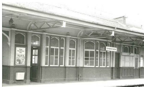
Platform waiting room with half-glazed door
