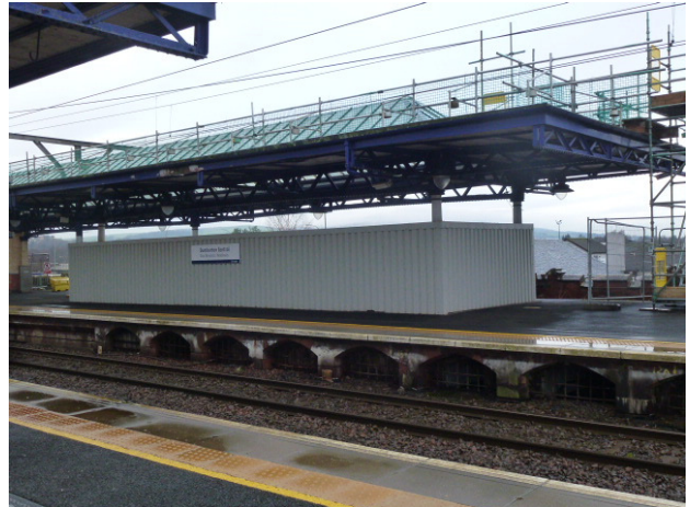
Figure 48 Stair enclosures and windows between platform and track
