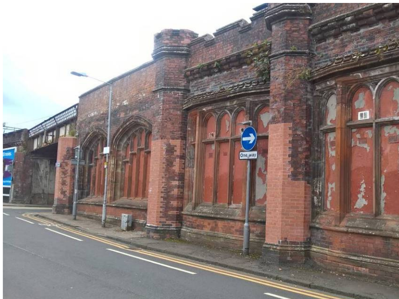
Figure 46 Bankend Road non-matching brick replacements and loss of detail at bridges
