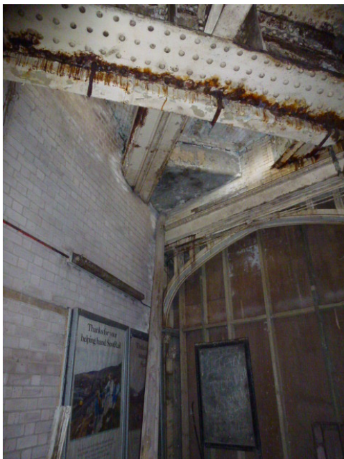
Corrosion in steel structure at foot of south stair
