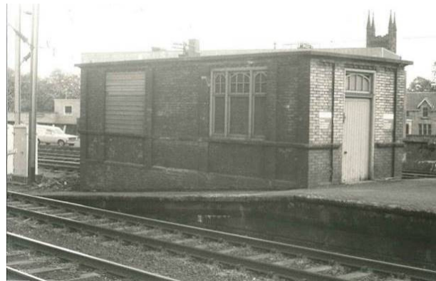
Figure 28 Mid-late 20 th century image of service building at end of the south platform. 75
