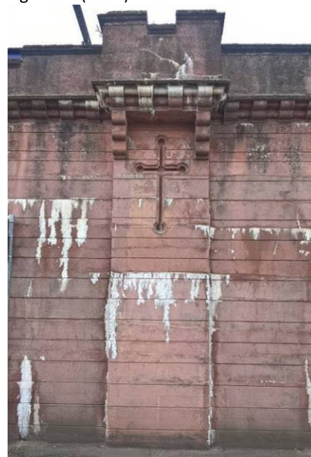
Efflorescence on north embankment walls
