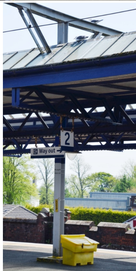
Figure 32 Electrification stanchions at top of access ramp (top) and on platform (bottom 81 )
