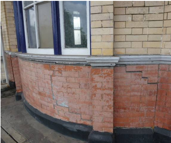
Figure 44 Platform buildings: showing movement, coating on brickwork, open joints, efflorescence, stone base, and drainage channel.
