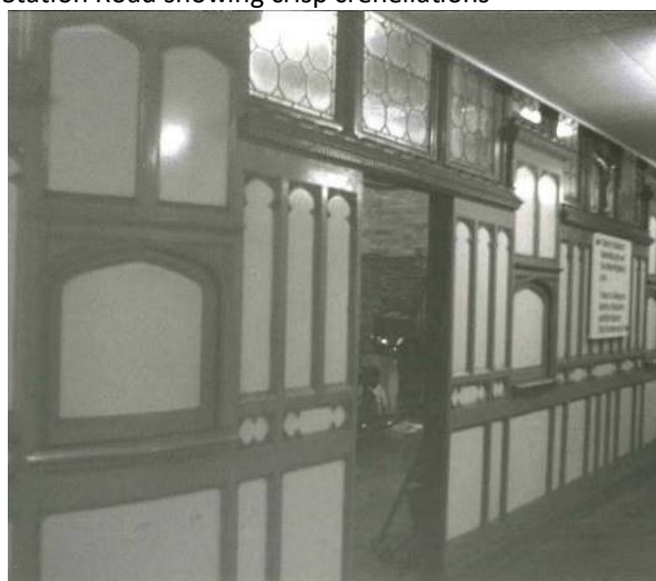
Timber screen to ground floor booking office
