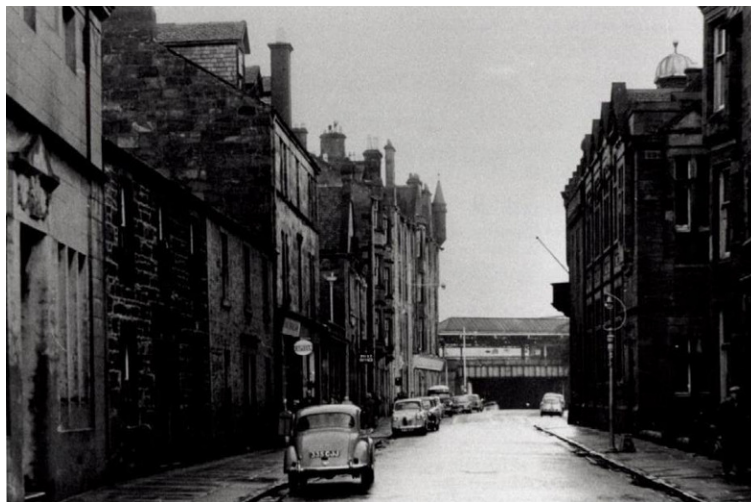
Figure 29 1965 photograph looking north along Upper College Street toward the station prior to roadworks and demolition. 76
