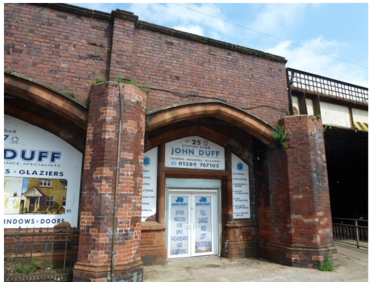
Figure 45 Inappropriate repairs - injected chemical DPC (L) and Non-matching brick replacements & loss of detail at Station Road (R)
