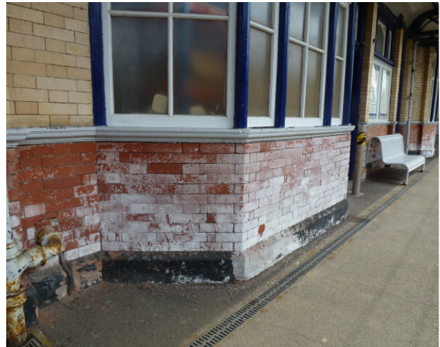
Figure 44 Platform buildings: showing movement, coating on brickwork, open joints, efflorescence, stone base, and drainage channel.
