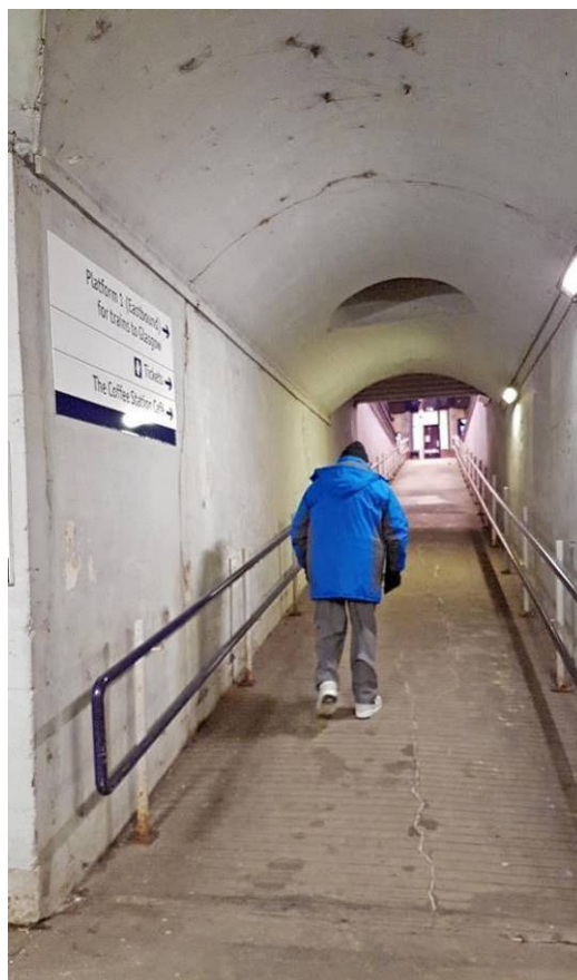
Figure 47 Access ramp and signage
