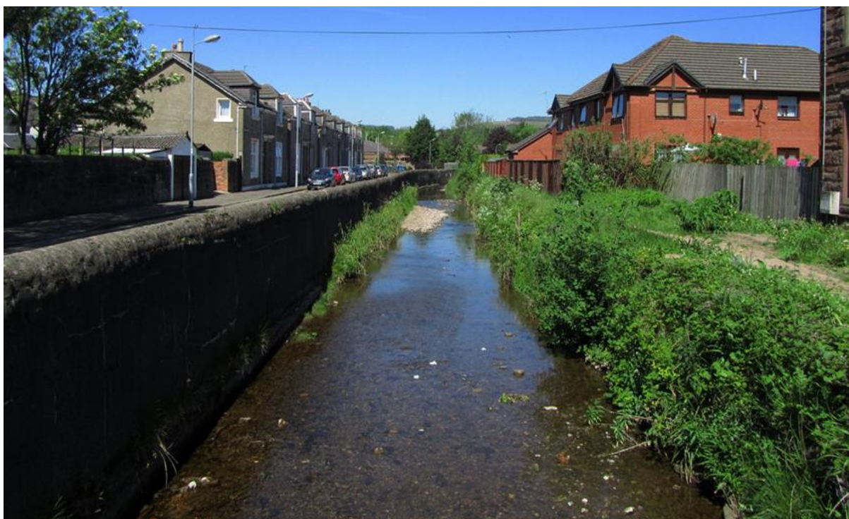
Figure 7: Existing flood wall at Buchanan Street (Source: Balfour Beatty)
