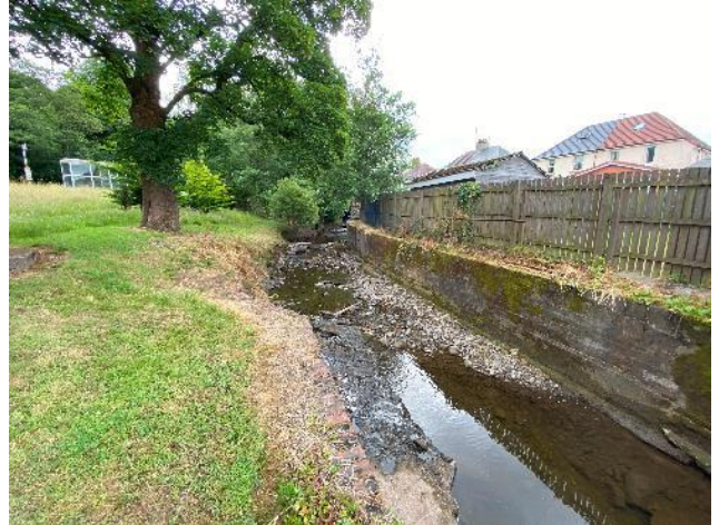
Plate 2: A view of the typical channel structure of Gruggies Burn between the A82 and Glasgow Road.
