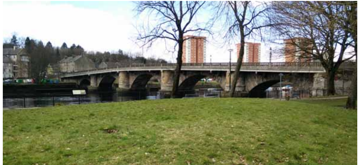
Old Dumbarton Bridge - Listed B
