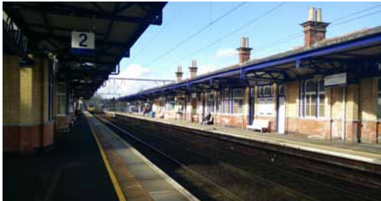
A-listed Dumbarton Central Station
