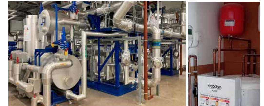
Photographs: Queens Quay Energy Centre and air source pumps
